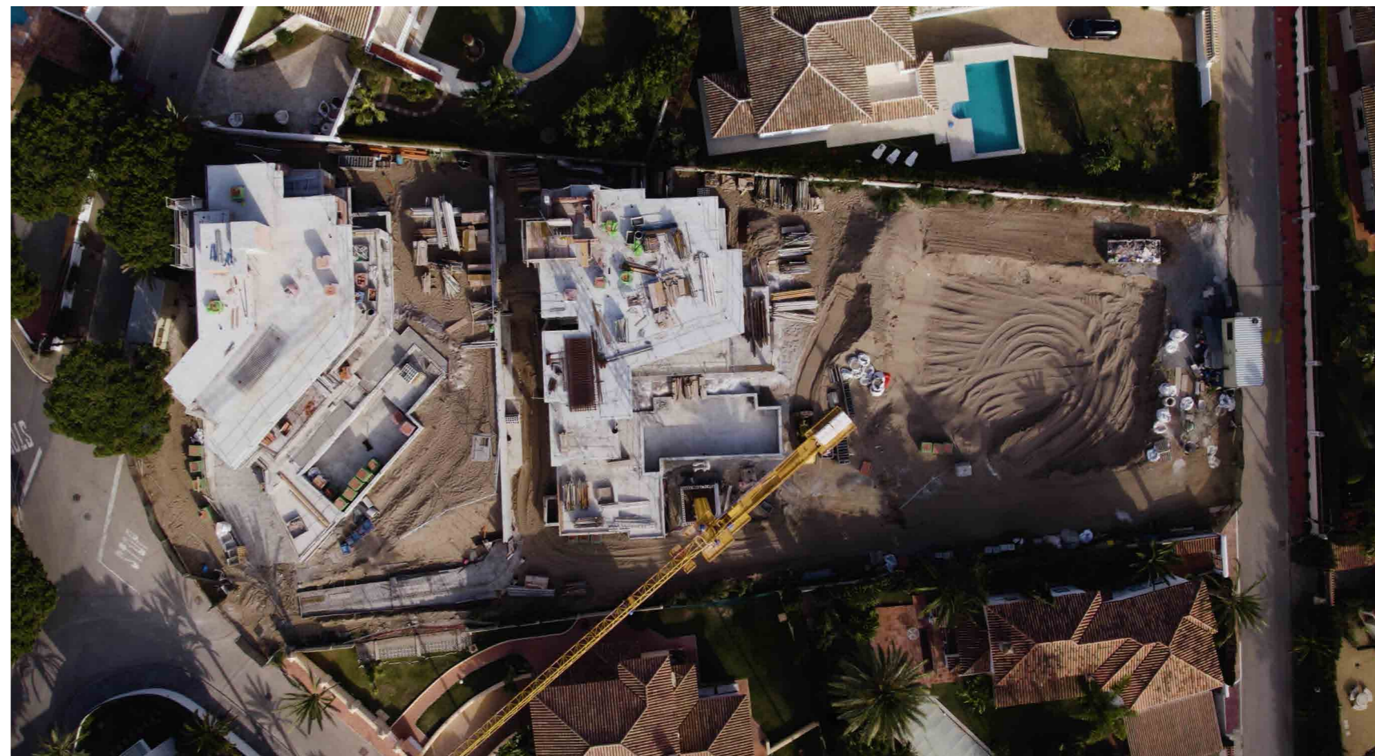
CONSTRUCTION SITE JANUARY 2022
