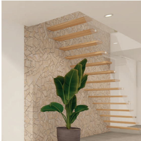
Interior staircase leading to first floor, cantilevered, with designer metal structure, with wooden steps.
